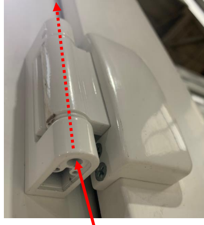
With grub screw suitably slackened off, gently tap pin out from underside off hinge with a suitable tool and remove pin from the top
