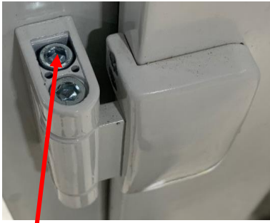
5mm Allen key gives + 4mm Height Adjustment (ON TOP OF HINGE) Replace cover caps when adjustment is finished
