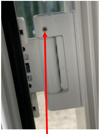
Open door to approx 90° to gain access to grub screw 2mm Allen key required- slacken off grub screw
